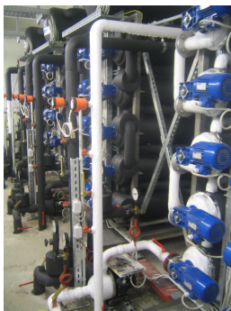
600 KW FLOW-ICE System Installation
