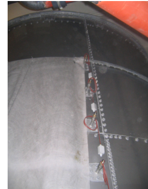
FLOW-ICE-System with 220m 3 thermal energy storage tank
